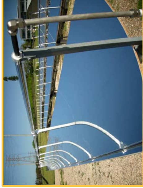
NEP Solar solution: continuous mirror surface
